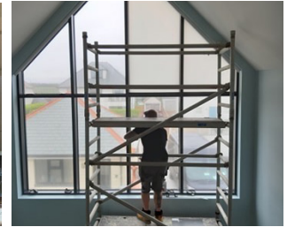
RETRO-FIT SWITCHABLE SMART FILM BEING INSTALLED ON YOUR GLASS
