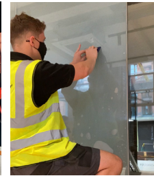
RETRO-FIT SWITCHABLE SMART FILM BEING INSTALLED ON YOUR GLASS
